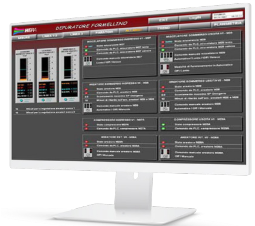
The data collected from the field is used to carry out a predictive control and therefore optimize machine use.
